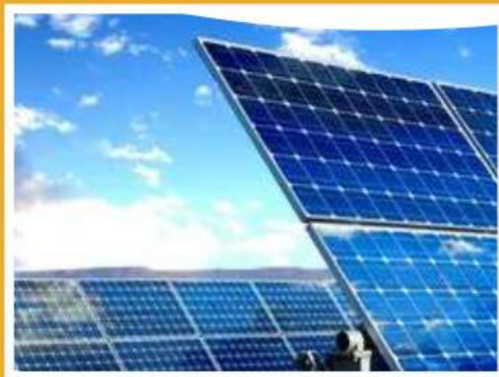
UP Solar Park-75 MW Parasan, Jalaun
